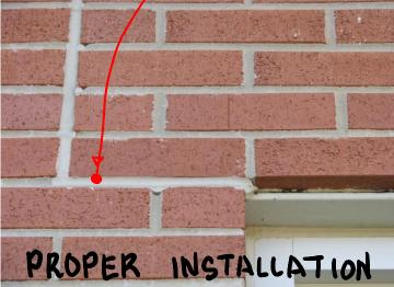
Mortar cracking occurs along the horizontal joint in front of the loose lintel. Sometimes we will see cracking down the face of the masonry and then over to the window opening, either in a horizontal pattern or diagonal.
