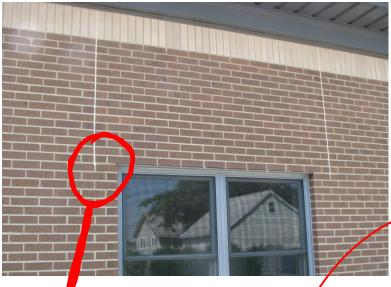
LOCATE A WEEP WITH-IN 4" OF THE END DAM.
